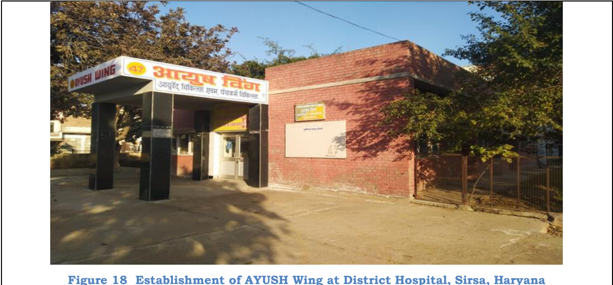
Figure 18 Establishment of AYUSH Wing at District Hospital, Sirsa, Haryana
